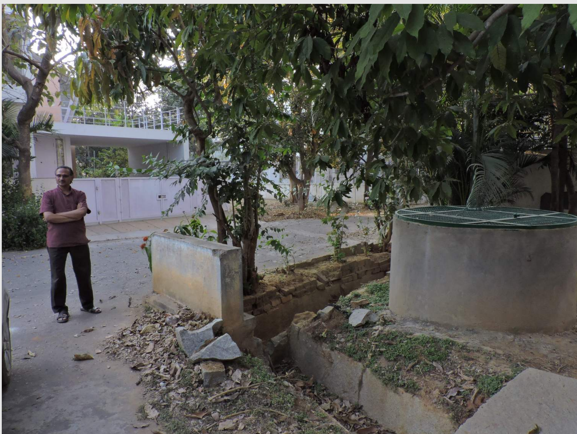
A water-harvesting tank in Rainbow Drive colony, Bengaluru, Karnataka.
