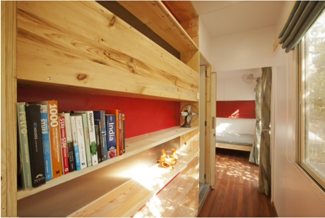
All the wood you see in interiors is used pine wood from packaging. One lamp and stools are made from discarded materials. Rest of the materials are new. Now in coming up similar container space project we are planning to utilise more reused materials.
